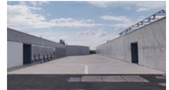
Data Center in Peltre (France)
