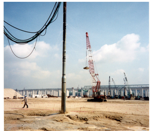
Pasir Panjang Container Terminal (Vibro Compaction)
