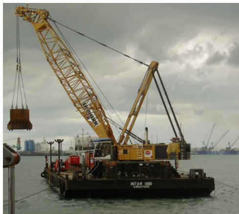
Pasir Panjang Phase 3 and 4 (Marine Dynamic Compaction)
