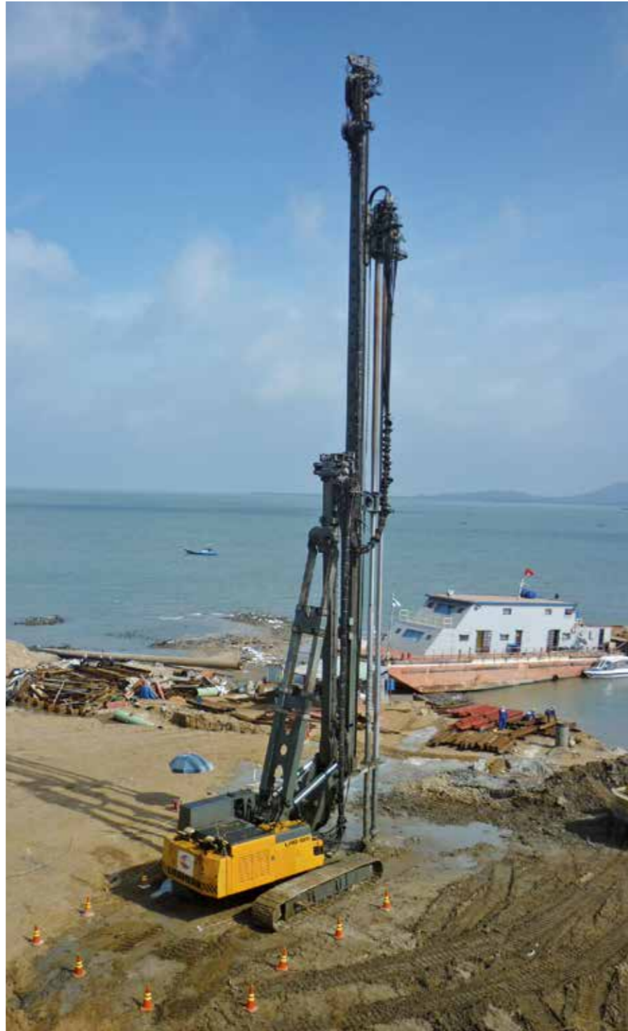
▲ Ground reinforcement of a Danish quay in Saigon, Vietnam
