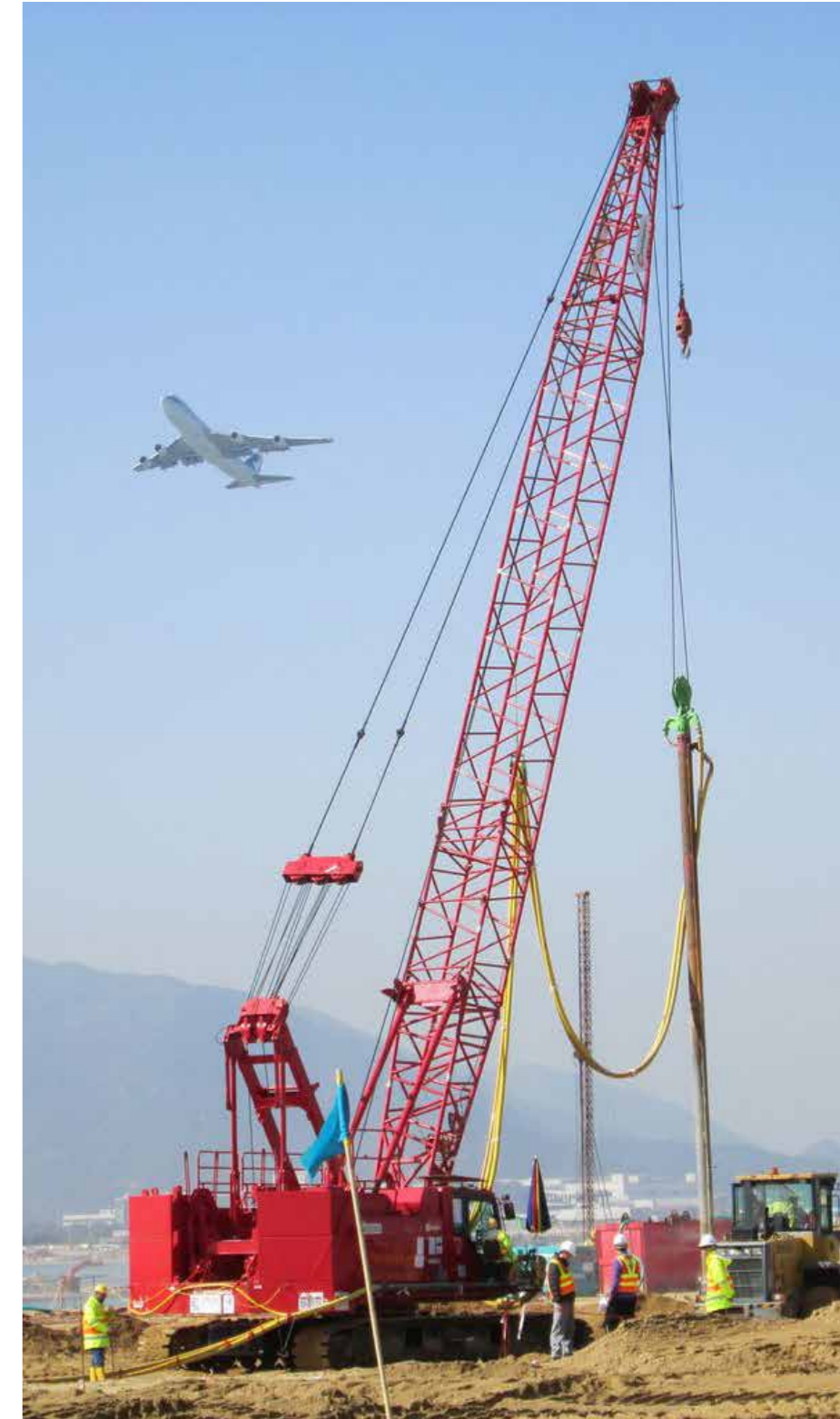
▼ Hong Kong Border Cross Facility
