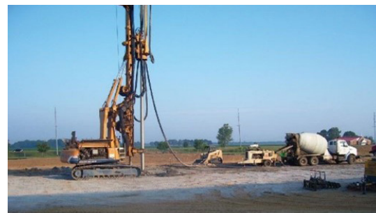
Unilever Ice Cream Freezer Warehouse (USA)
