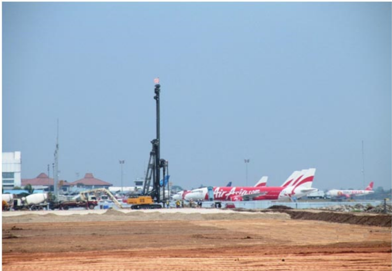
Figure 1: View of Terminal 3 Soekarno Hatta International Airport – Soil Improvement Works Ongoing
