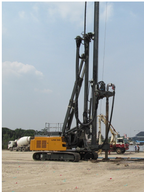
Figure 2: CMC Equipment - Liebherr LBR155
